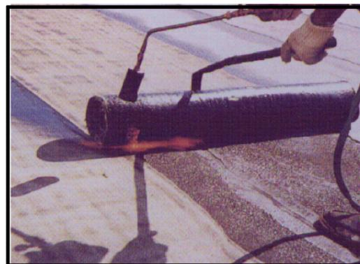
**EABASSOC APP Torching Membranes** are applied in the waterproofing of flat or pitched roofs, either as a single layer system or as the top layer in a built up roof. They are compatible with a wide array of deckings and roofing and insulation products. They can, therefore, be applied both in new constructions and in renewal work.
