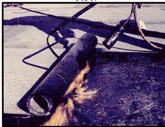
**EABASSOC SBS Torching Membranes** are applied in the waterproofing of flat or pitched roofs, either as a single layer system or as the top layer in a built up roof. They are compatible with a wide array of deckings and roofing and insulation products. They can, therefore, be applied both in new constructions and in renewal work.
